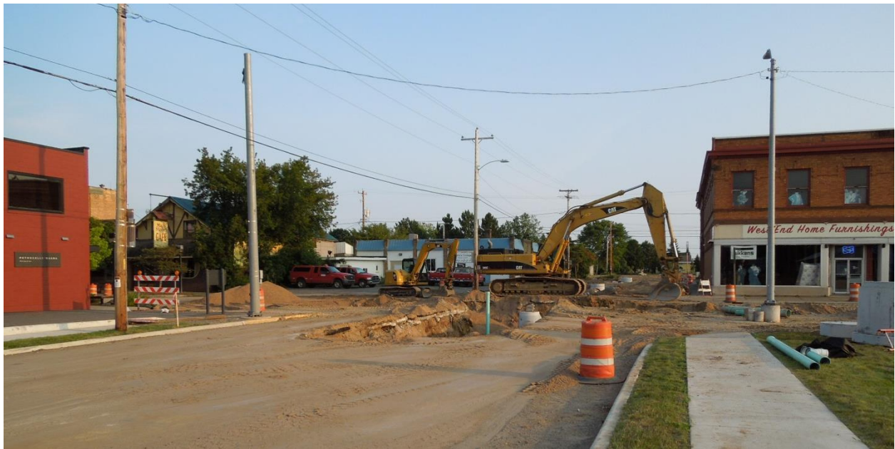
Street reconstruction funded by a 2013 Downtown Infrastructure Grant
